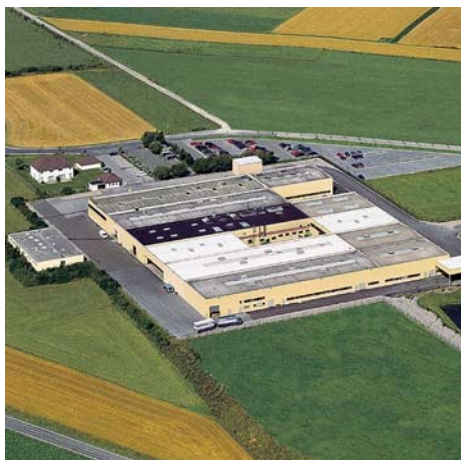
Production facility in Brilon
